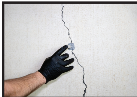
02: Press injection port firmly directly over the crack
