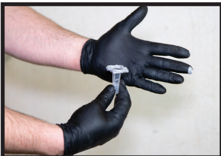
01: Roll the injection port in BARRICADE™ CONCRETE REPAIR CRACK PREP SURFACE PASTE
