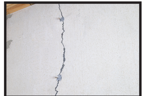
03: Cover over previously marked locations
